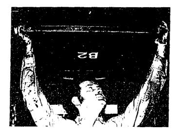
FIG. 30. REMOVAL OF BELLYPAN PANELS.
